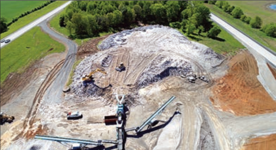
In the median of Interstate 24 in Trigg County, this repurposing facility is crushing previously used sections of the interstate and making aggregate for new work.
